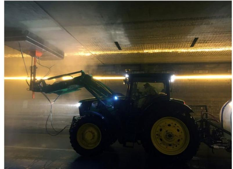
*Metro District's tunnel washer is mounted on a John Deere tractor. The washing equipment can be removed, freeing the tractor up for other duties. This photo was taken during a cleaning of the Lowry Hill Tunnel on Oct. 21. Photo by John Bleniek*
