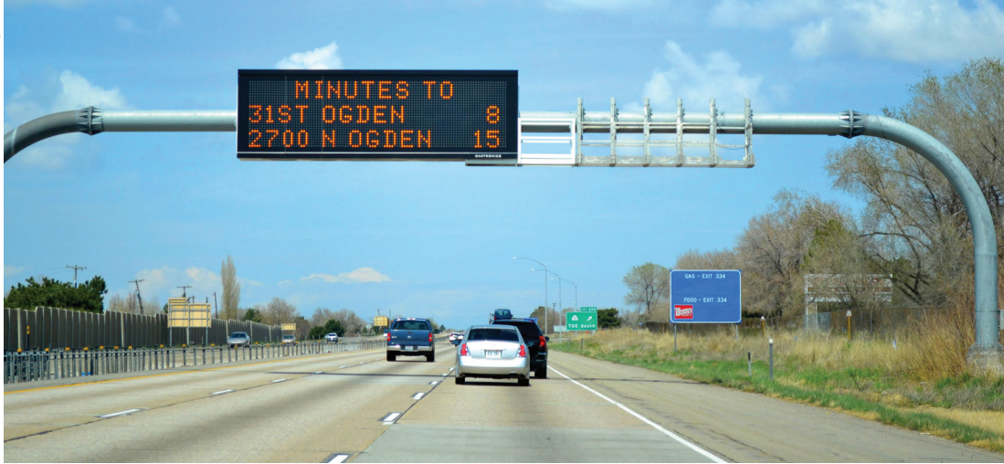
Variable message signs—an example of an early technology developed from transportation research—now are standard highway features.
