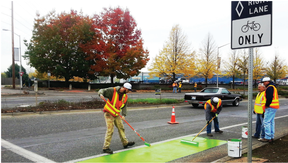
Washington State Department of Transportation (DOT) workers paint bike lanes green. The agency has used the process presented in NCHRP Report 803: Pedestrian and Bicycle Transportation Along Existing Roads , throughout the state.
