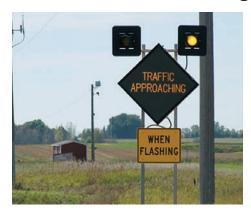
**TRAFFIC & SAFETY** – MnDOT has installed systems at more than 50 rural locations to alert drivers approaching stop signs on minor roadways when traffic is approaching on a major roadway. Researchers evaluated the effectiveness of these life-saving systems to help determine when and where to deploy additional systems. Drivers were 50 percent more likely to come to a complete stop at intersections where such a system was present.
