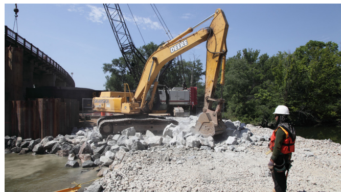
If properly designed, inspected, and maintained on a regular basis, riprap placed around bridge piers can provide long-term protection against scour. (Image courtesy Virginia DOT)
