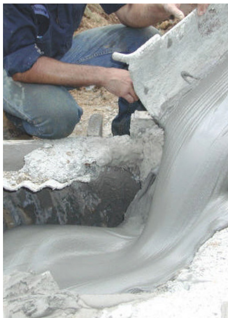
Flowable fill is self-leveling and self-compacting. It requires less labor than traditional fill materials.
