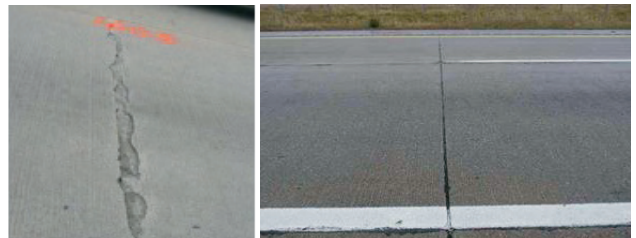
Sections of US-23 test road: (left) Typical transverse mid-panel crack spalling in Section B (blast-furnace slag aggregate) in 2006. (right) A typical transverse joint found in Sections A through E in 2016. There was no sign of deterioration at the joints.
