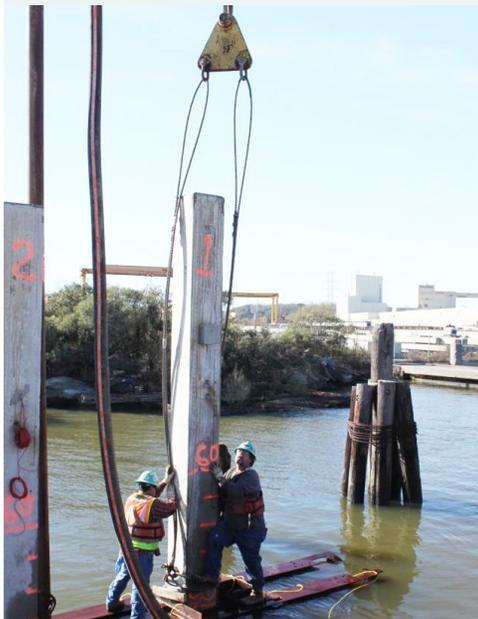
Marine environments can be highly challenging for concrete bridges with the salt from ocean water corroding steel reinforcements in their foundations. After 11 bridges in coastal Georgia were found to have remaining service lives of only 24 to 58 years, Georgia DOT investigated replacing conventional steel in prestressed concrete piles with stainless steel alloys.
