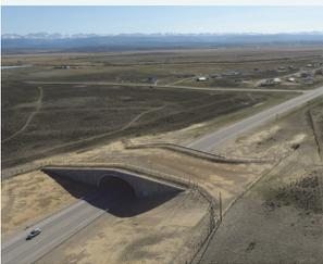
Wyoming research keyed in on employing the right highway crossing solutions for the right species. Wyoming DOT installed six underpasses and two overpasses along a state highway and undertook a three-year study to track movement of two large species with different movement patterns: mule deer and pronghorns. Researchers found 79 percent of mule deer moving from one side of the highway to the other used the underpass, and 93 percent of pronghorns used the overpass.
