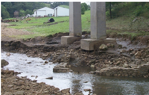
NCHRP Projects 24-07(2) and 24-23 developed comprehensive guidance for countermeasures to bridge scour, a leading cause of highway bridge failures.
