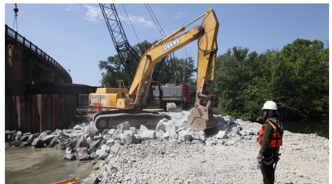
If properly designed, inspected, and maintained on a regular basis, riprap placed around bridge piers can provide long-term protection against scour. (Image courtesy Virginia DOT)
