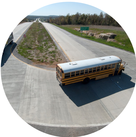
Traffic engineers at the Missouri DOT are leading implementation of the J-turn intersection, an innovative median treatment highlighted in NCHRP Report 650.
