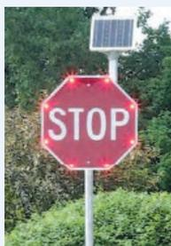
Flashing LEDs improve the visibility of stop signs, causing some drivers to reduce their speed when approaching them.
