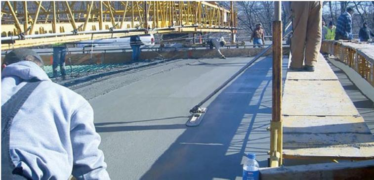
This project provided extensive testing of crack-reducing construction techniques, materials and mix design strategies. The tests validated several strategies that MDOT is already using and helped the department eliminate poorly performing mixes.
