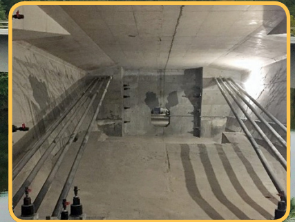
Reinforcements: Steel cables inside the box bridge add strength.
