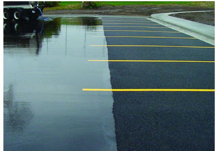
Porous asphalt pavement (at right, side-by-side with standard pavement) easily handles runoff in a parking lot. (Image courtesy of NAPA)
