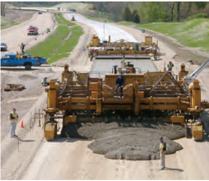
Built for the long haul in Wisconsin: Motorists can expect long pavement life thanks to advances in materials testing and construction. (Image courtesy of Wisconsin DOT)
