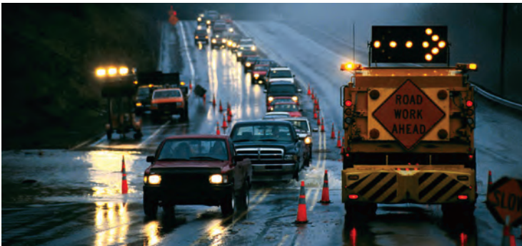
NCHRP and AASHTO together address safety challenges such as those presented by road construction, nighttime driving, and poor weather. (Image courtesy of FHWA)
