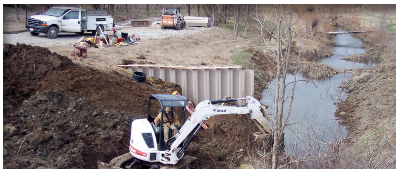
Downstream wetland restoration is an off-site BMP that can be used as part of a watershed-scale approach to mitigating pollution impacts from construction activities.
