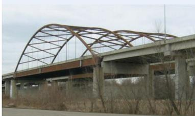
The Cedar Avenue Bridge is a steel tier-arched bridge over the Minnesota River, chosen because it is fracture-critical but has no history of cracking.
